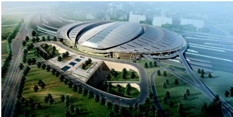
The new Beijing South Railway Station from the air. The solar modules from Würth Solar traverse the center of the station roof like a ribbon in a chess board pattern with alternating clear glass arrays. (Computer simulation. Source: Ruihua Construction Corporation)
