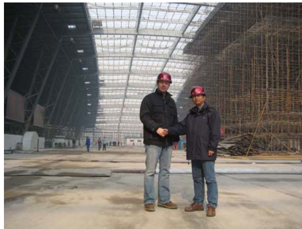
Timo Bauer (l.), product manager at Würth Solar, and Landrew Zhou (r.), Vice President Ruihua Construction Corporation (RHC), at the construction site of Beijing South Railway Station. Completion in August 2008 (Source: Würth Solar)
